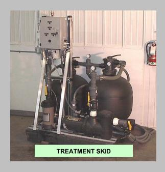
Clarified water is pumped to a treatment unit where it is treated with granular activated carbon. Oxidation is provided as a polishing step where needed to meet treatment or recycle objectives objectives.
