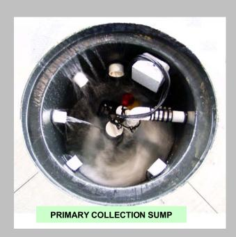
Dirty wash water collects in the primary sump. At water high level, the pump engages. During pumping, the water is vigorously agitated to ensure that grass, and dirt, do not accumulate in the sump.
